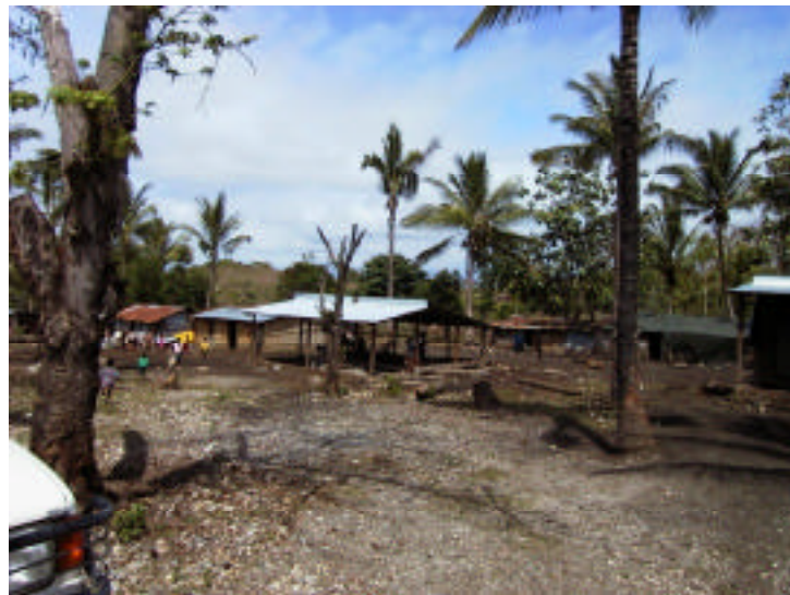
Shelter Construction at Hatahoudo
